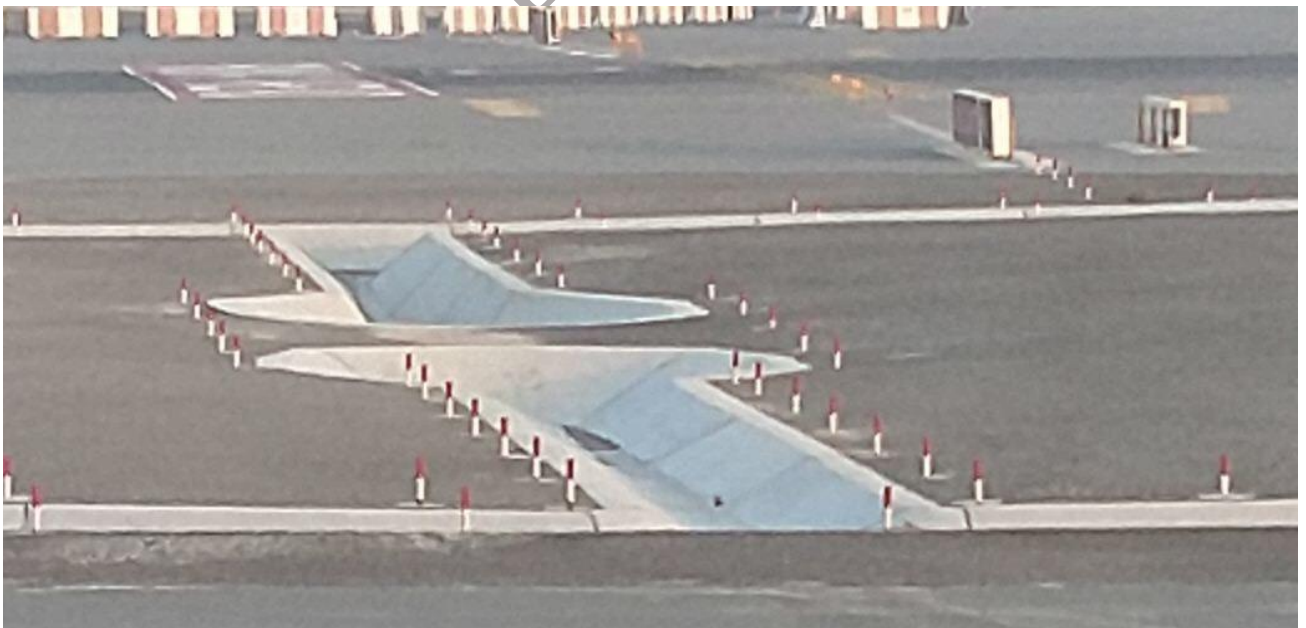
Drains at Dubai Airport with Marker poles
