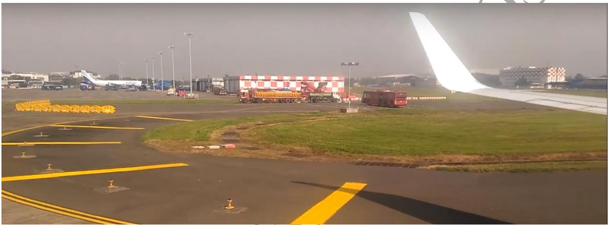
Drains covered with Steel Grills at Mumbai Airport
