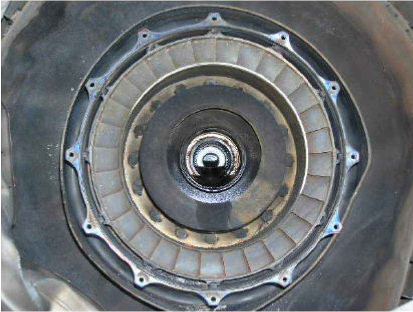
Small exit duct and compressor turbine guide vane ring, in-situ.
