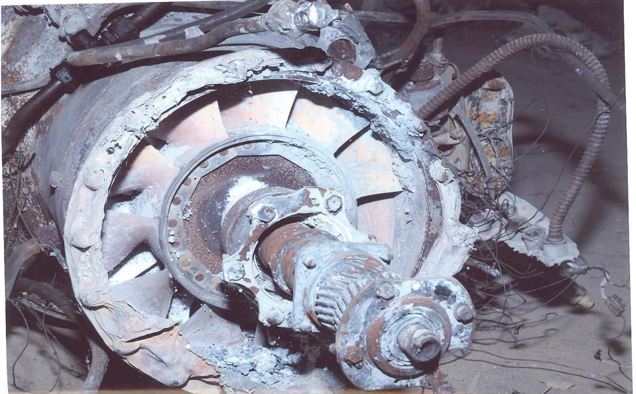
Fig. 12 Inlet to 1st Stage Compressor
