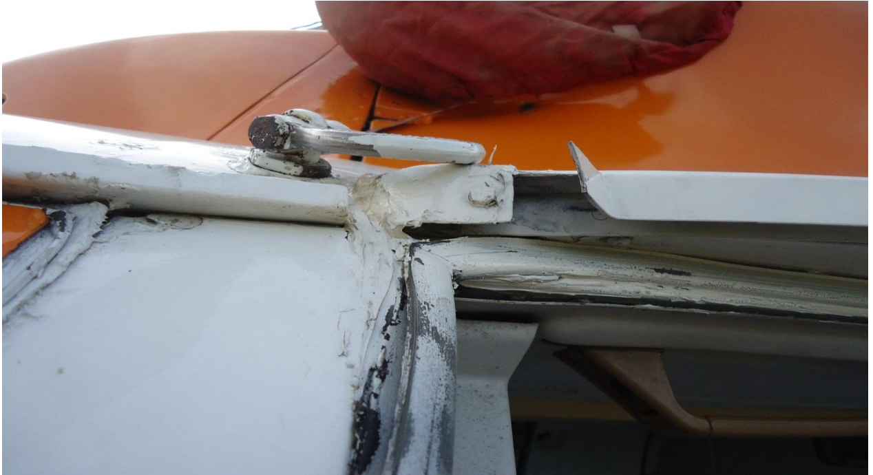
1. Portion of LH sliding door Upper Rail had a tear near the forward end.
