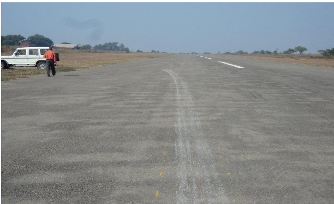
Fig.4 Showing deep cut due propeller blade strike on the runway
