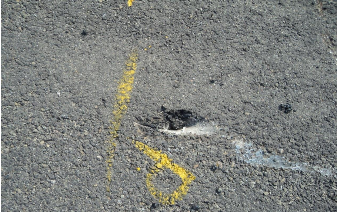
Fig.4 Showing deep cut due propeller blade strike on the runway
